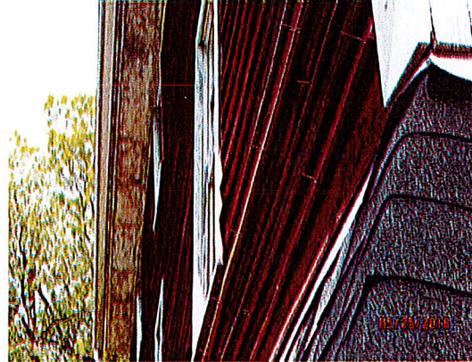
Fasteners coming out at South elevation
