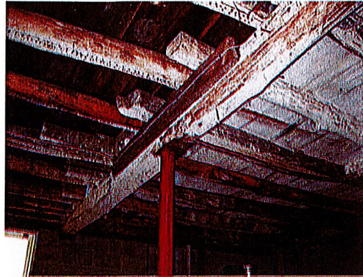
Basement column connection
