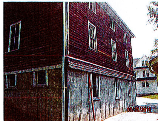
Cedar siding falling off South elevation (a piece is leaning against foundation in photo)
