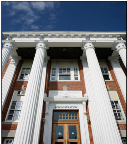
WSU Administration Building entrance
